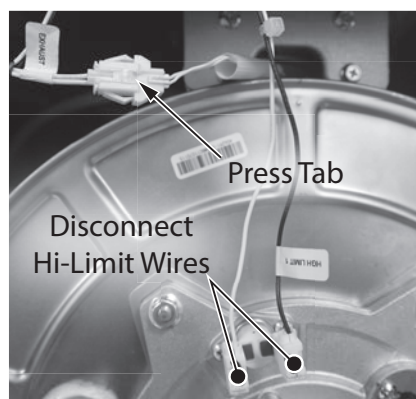
Figure 143 - Disconnect hi-limit and exhaust thermistor wiring
