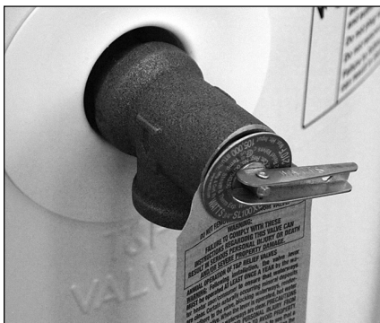
Figure 25 - Temperature and Pressure Relief Valve
