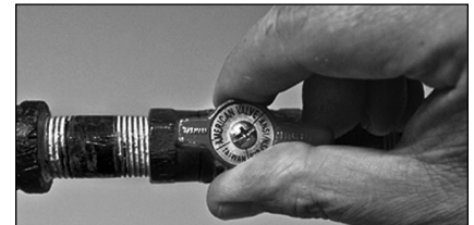
Figure 58 - Gas valve in “on” position.
