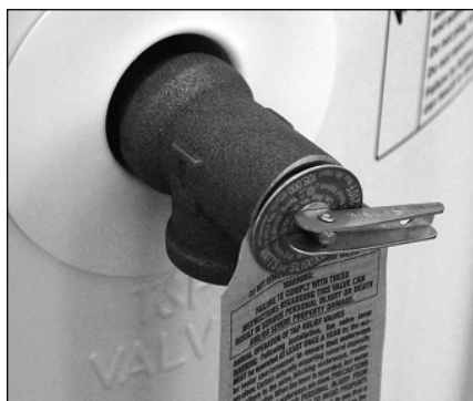
Figure 25 - Temperature and Pressure Relief Valve
