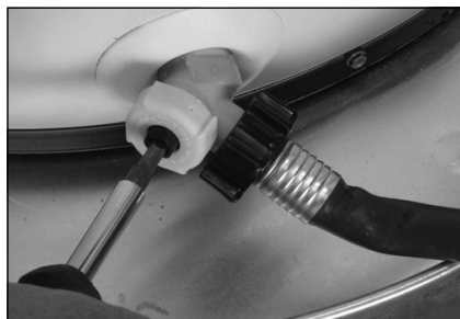
Figure 20 - Draining the old water heater.
