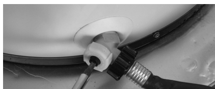
Figure 26 - Drain Valve
