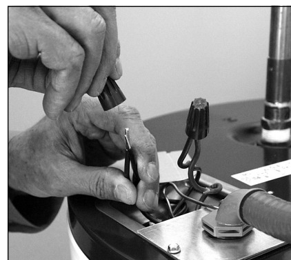
Figure 19 - Connecting the electrical wires.
