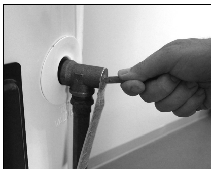
Figure 38 - T&P Relief Valve
