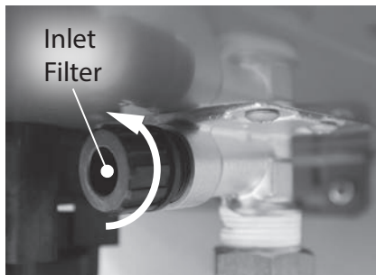
Figure 23 - Removing the inlet filter
