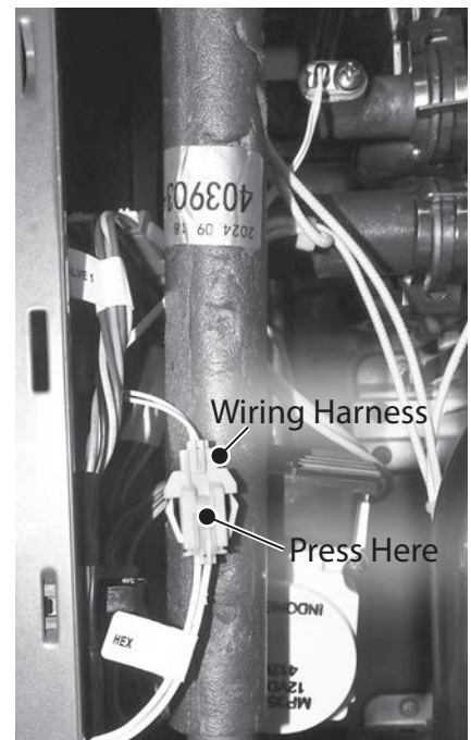
Figure 76 - Wiring harness location
